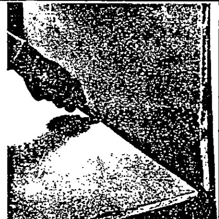
With the partially broken portion folded back, cut the exposed backing paper from above or by an upward stroke from below.
